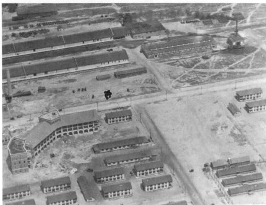
Early construction at Fort Benning—29th Infantry Barracks, circa 1924. ( U.S. Army Collection, National Archives )
